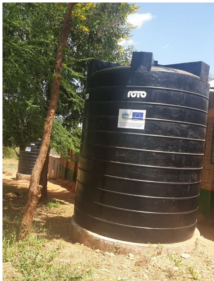
Water storage tanks at Cieria Primary School.
