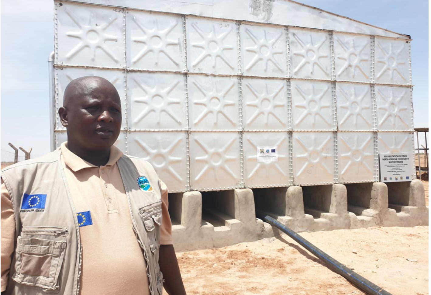
NDMA Isiolo County Drought Coordinator Mr. Lordman Lekalkuli at the 231,000 litres booster tank near Mata Arba village. The steel tank is part of the Merti-Korbesa Water Supply Project.
